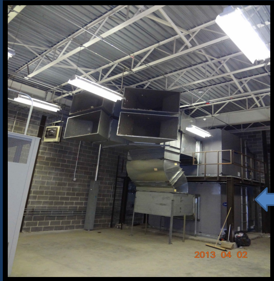
Existing roll filters to be replaced with filter rack & cartridge filter
